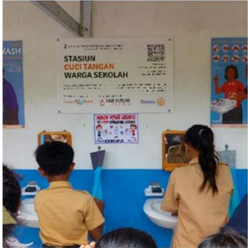
ABOVE: The supply of clean water, toilets and septic systems, medical supplies and health education materials have been a revolution for Sumba's small village centres. Hand basins installed at schools encourage all students to wash their hands.
