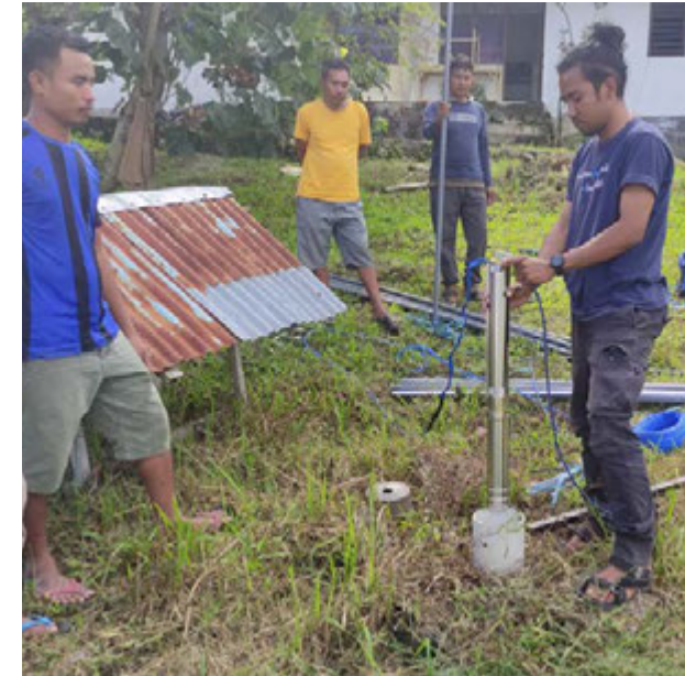
Submersible pump installation
