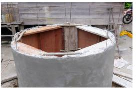
In the first week, the Wai Maringu group's construction of the ferrocement water tank reached the second layer of plastering on the inside. The process progressed quickly thanks to the active participation of the community, who worked together until late at night, and favourable weather conditions, ensuring smooth and efficient work.
