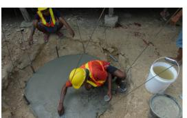
The first week focused on material distribution, site clearing, foundation assembly, tank mold installation, interior and exterior plastering, and pipe installation.
