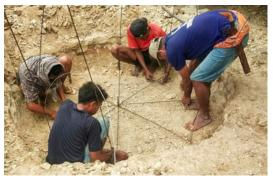
Construction of the second ferrocement water tank commenced on June 5, 2025, and within four days, it had reached 70% completion. The stages included site clearing, foundation construction, installation of the mall and reinforcement, and exterior plastering. A parallel work strategy and active community participation accelerated the process.
