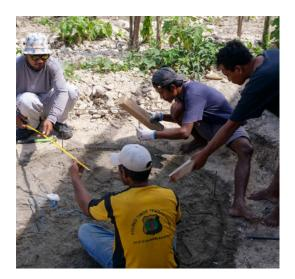
Construction of the ferrocement water tank in Wai Pandulang has reached approximately 90% completion, including material distribution, formwork installation, plastering, and piping installation.
