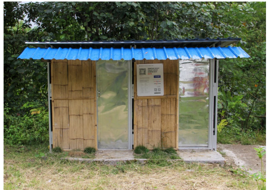
An example of a picture of a healthy sanitation building that we have previously built in Mbinu Dita village
