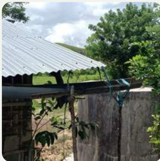
Rainwater Harvesting in Teacher's Mess
